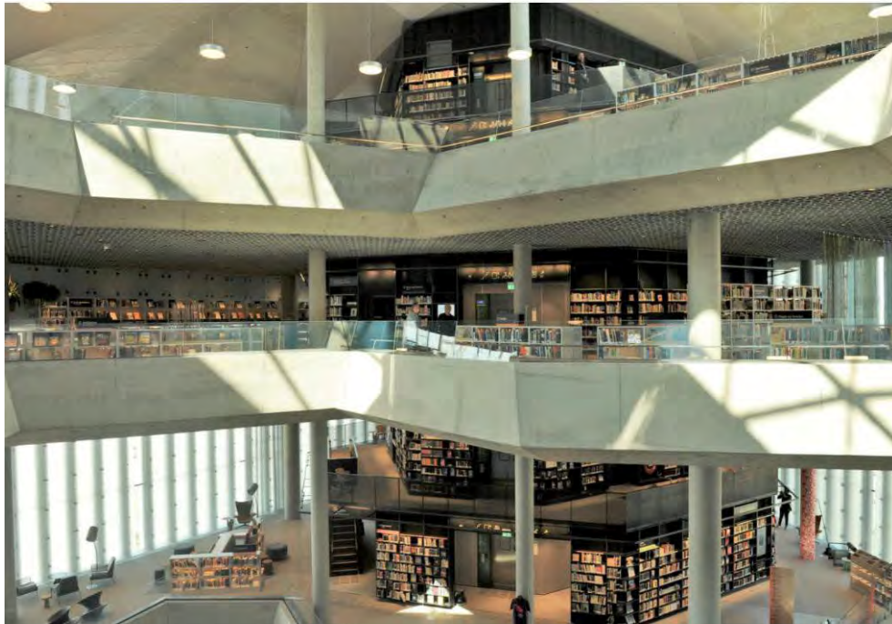
The Deichman Bjørnvika library in Oslo has six floors held up by three towers, leaving an open atrium at the building's center. It was named public library of the year in 2021. (Sigrid Harms/picture alliance via Getty Images)
